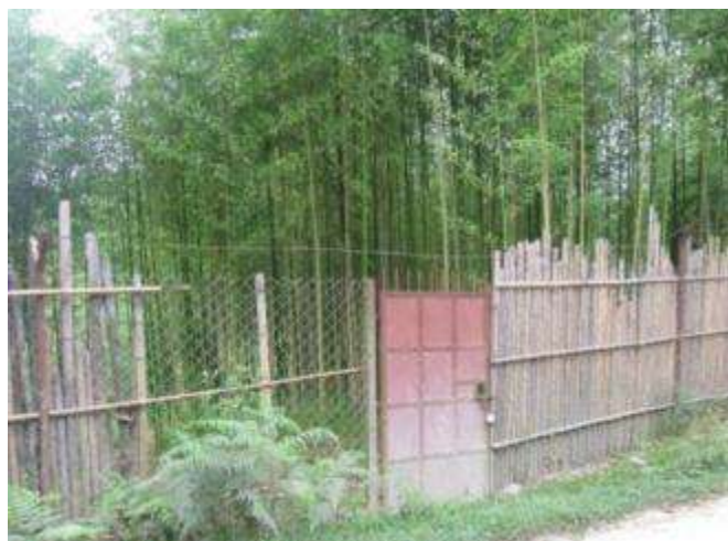
Improved fencing of Bamboo Plantation with Iron grided gate for protection
